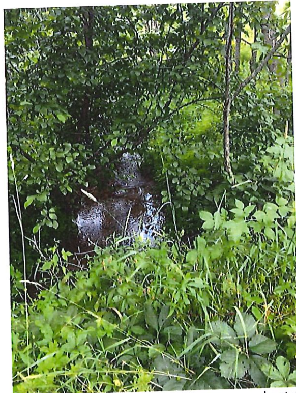
Photo 11. Looking downstream at stream culvert along farm lane.
