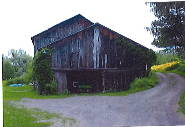
Photo 15. E side of barn.
