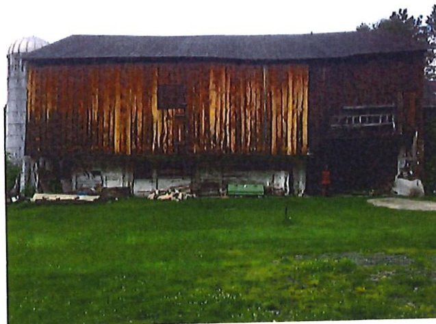
Photo 16. South side of barn.
