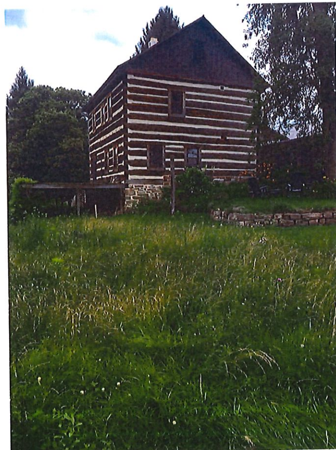
Photo 24. E side of the house.
