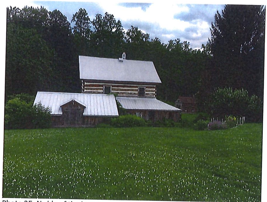
Photo 25. N side of the house.
