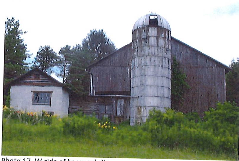
Photo 17. W side of barn and silo.
