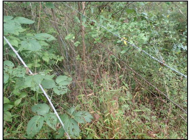
Evidence of property boundary with old woven wire fence (Southern Line Stand 3)
