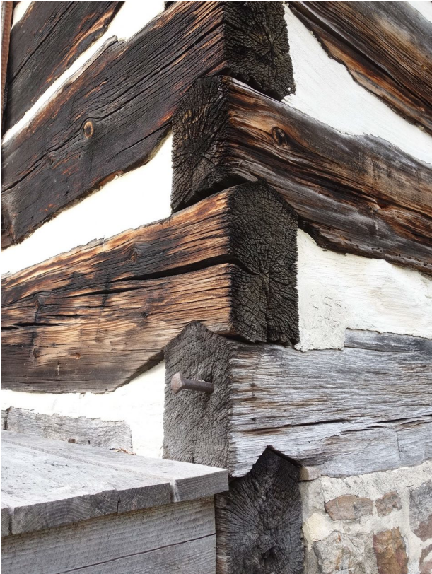
Details of south-east corner logs, bottom logs oak, others pine
